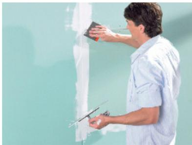
Spackle the groove in accordance with the directions of the plasterboard and filler manufacturers.
