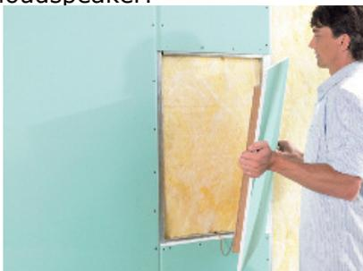
Place the loudspeaker in the prepared recess. In order to achieve an optimum bond between the AmbientTone loudspeakers and the smoothing cement, please observe the directions of the filler manufacturer with regard to edge preparation of the plasterboards you want to spackle. (e.g. folding of the edge where the speaker is inserted)
